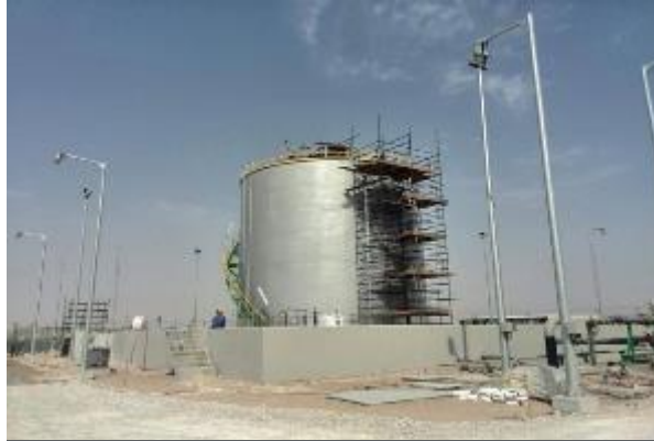
Fabrication of water storage tanks
