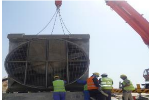
Cooler Erection
