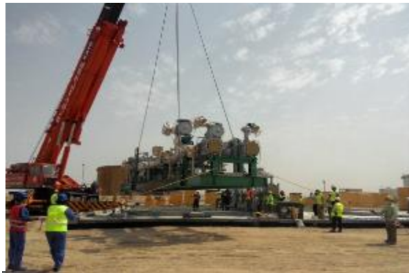
Installation of metering skid
