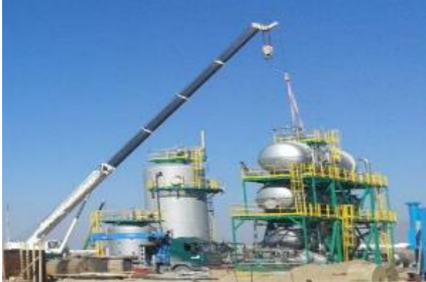
Produced Water Vessel Installation
