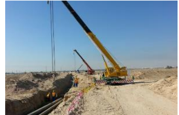
Off-plot pipe laying
