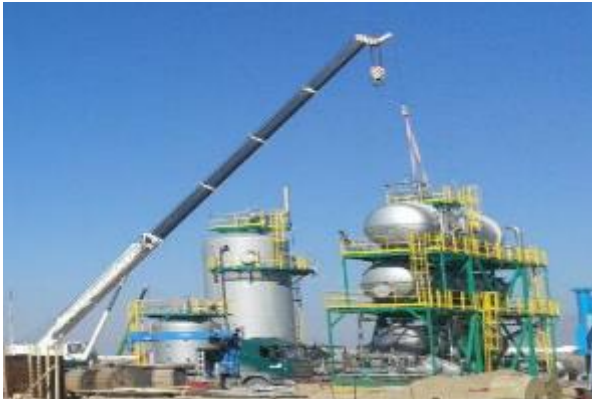
Produced Water Vessel Installation
