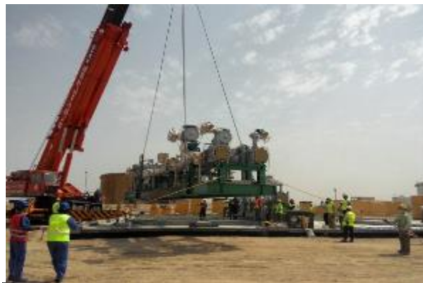
Installation of metering skid
